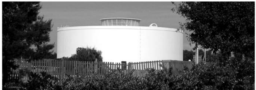
SOUTHLAKE UTILITIES, INC. 1.0 MG SELF-WASHING WATER STORAGE TANK WITH 5000 GPM AERATOR CONSULTING ENGINEERS: SAMBAMURTHI MUNIPALLI, PE
