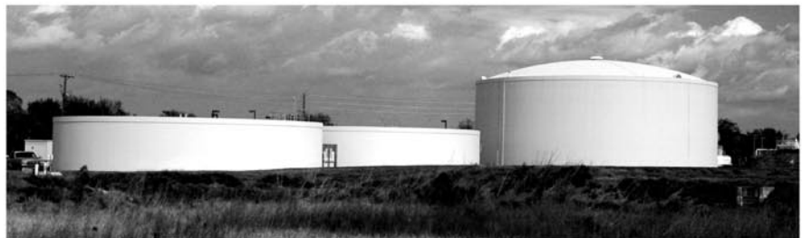
SARASOTA COUNTY - VENICE GARDENS WRF 3.0 MG EFFLUENT WATER STORAGE TANK & TWO - 0.7 MG DIGESTERS CONSULTING ENGINEERS: POST BUCKLEY SCHUH & JERNIGAN, INC.
