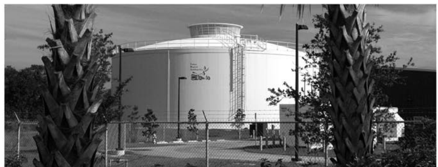
CITY OF KISSIMMEE 2.0 MG WATER STORAGE TANK WITH 12,000 GPM AERATOR CONSULTING ENGINEERS: JACOBS CIVIL, INC.
